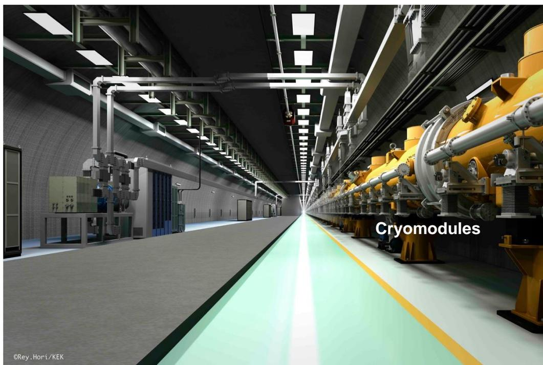
Figure 2.8. An illustration of the inside of a main linear accelerator tunnel (shield walls are not shown).
