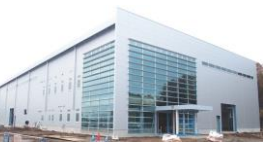
KEK Cryomodule Facility COI building
